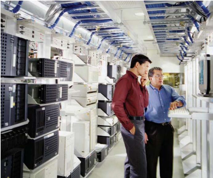
The Tellabs 5500 NGX-S switch simplifies service delivery and helps reduce operating costs.
